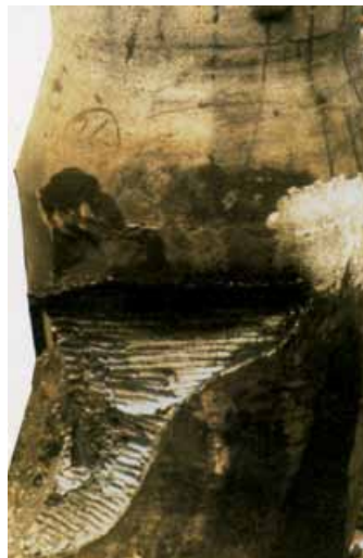
Steam chest casting showing large area removed by thermal gouging
