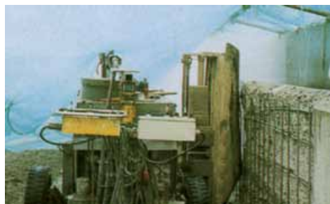
Robot machine water jetting a bridge side wall
