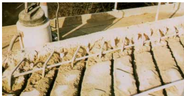
Concrete surface after water jetting
