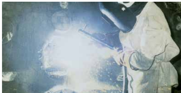
Air-carbon arc gouging in process
